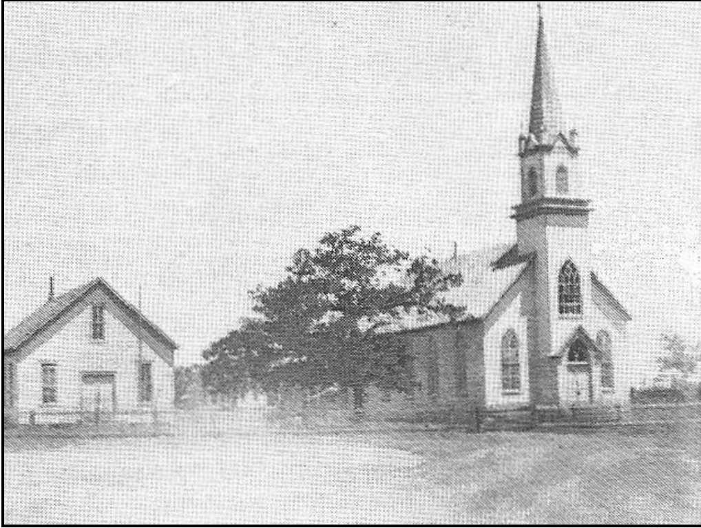
The school was finished near the end of 1906.
